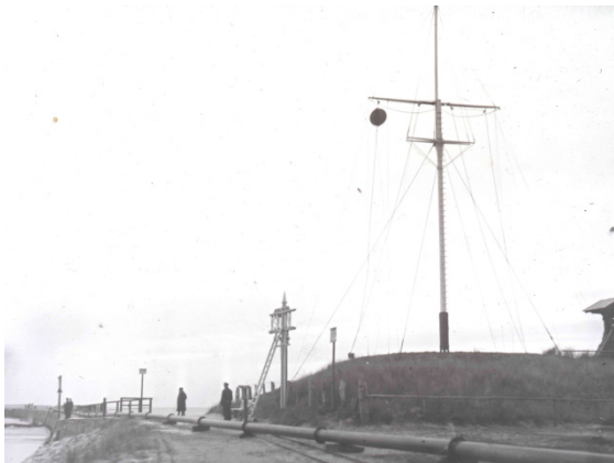
Figure 1. Signal station in Leba (Poland). Optical signals are balloons, triangles, cylinders and flags (source: DWD, archive of the German Naval Observatory Hamburg).
