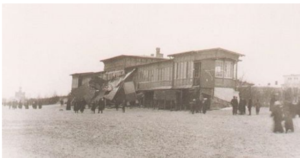
Figure 3: Postcards showing damages of the Beach Hall in Dziwnów caused by the storm surge on December 30, 1913. [1]
