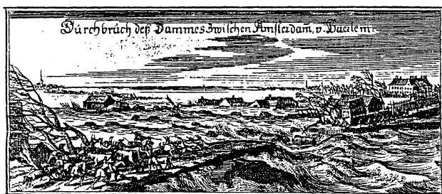
Fig. 1 Historical engraving of a storm surge with dyke failure in the Netherlands in 1673
